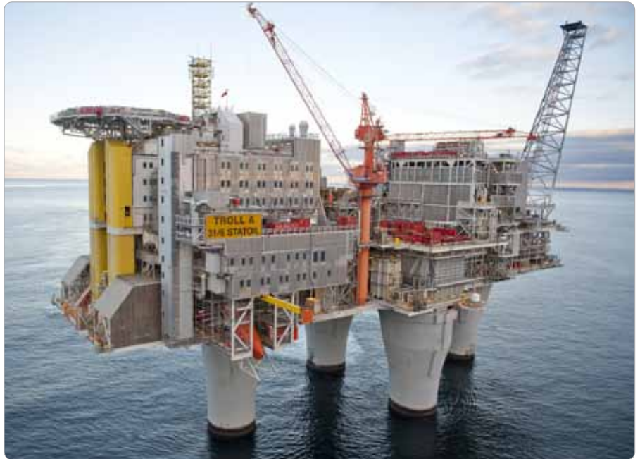
...offshore oil platforms... (Troll A platform, Statoil / Photo Øyvind Hagen).
