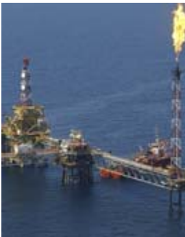
IECEX certification covers offshore oil platforms...
