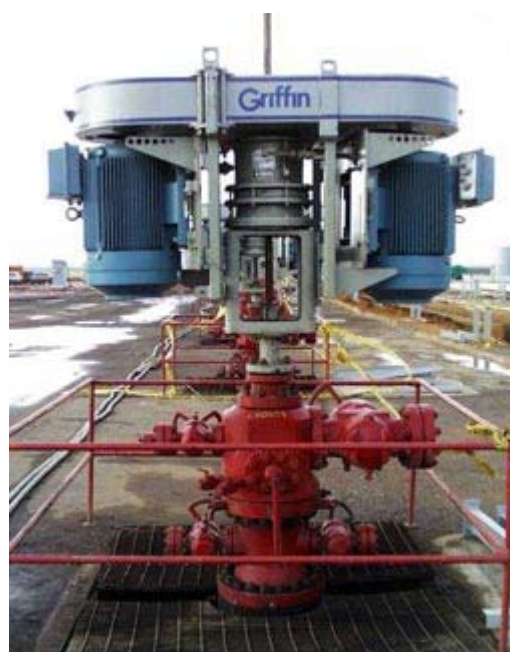
This Progress Cavity Pump, used for pumping heavy crude oil, is driven by two ABB motors.
